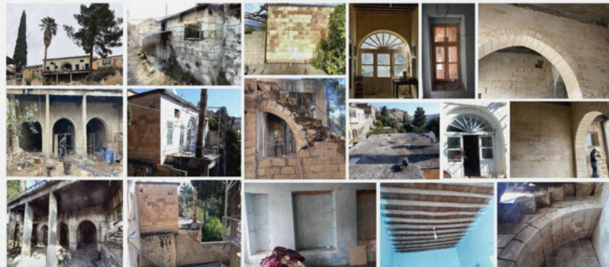
Halfeti Civil Architecture: Mirkelam Houses Restoration Project – Before Application
