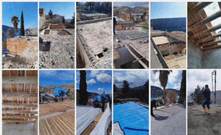
Halfeti Civil Architecture: Mirkelam Houses Restoration Project – Roof Applications
